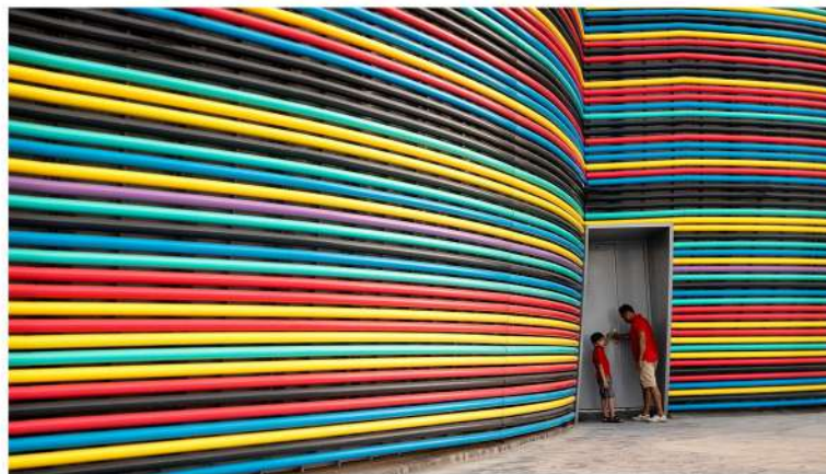
NPS eHM Thirumalai Ganesh Sheerapathi (United Arab Emirates) Optical Cable Cabin
